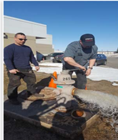
Utilities Maintenance personnel performing routine fire hydrant flushing.
