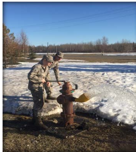
Utilities Maintenance personnel performing routine fire hydrant flushing.
